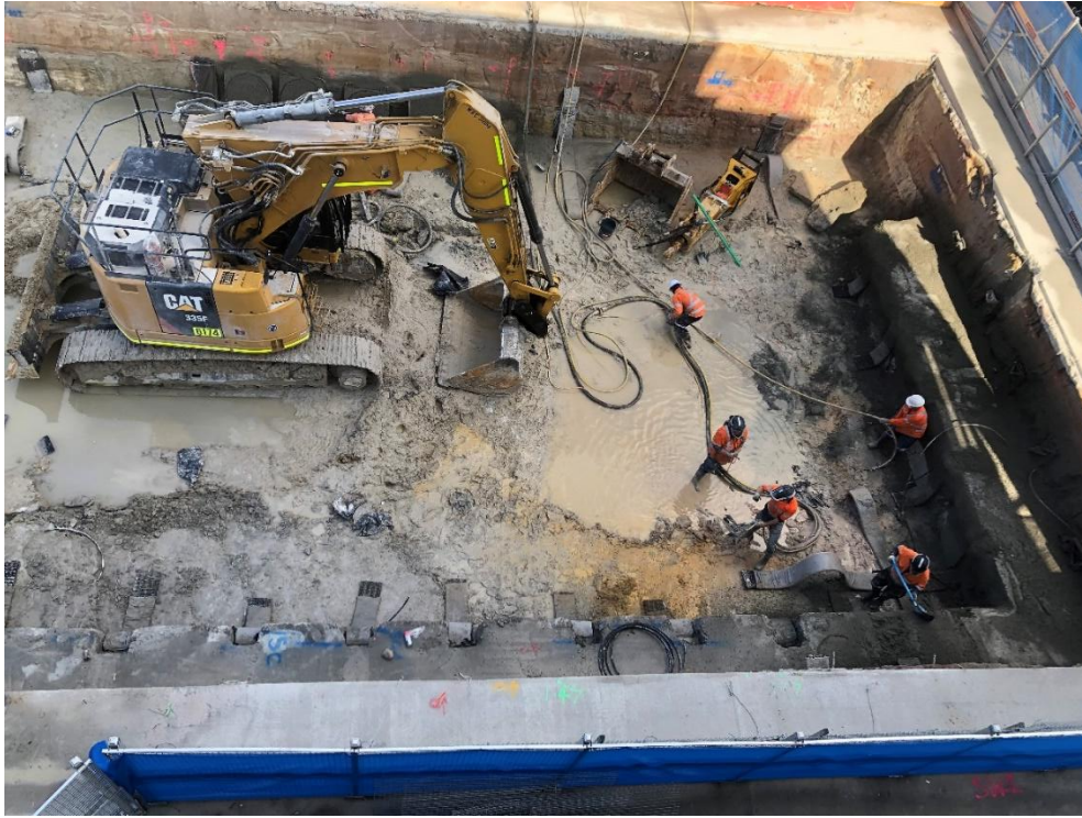
Figure 4. Hand spraying Shotcrete
