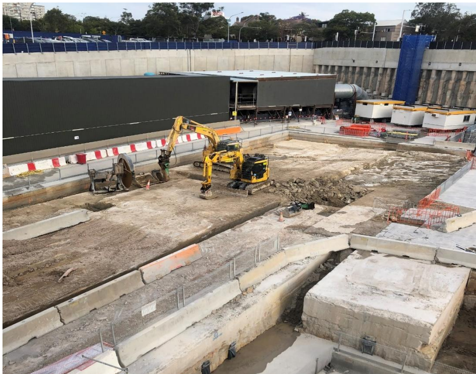
Figure 10. Hammering and mucking out trenches for building footings
