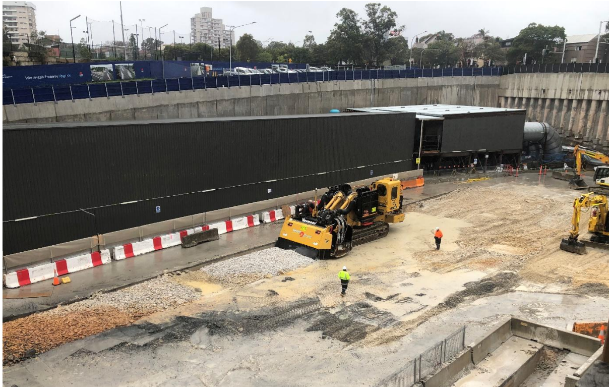
Figure 8. Surface miner excavating material
