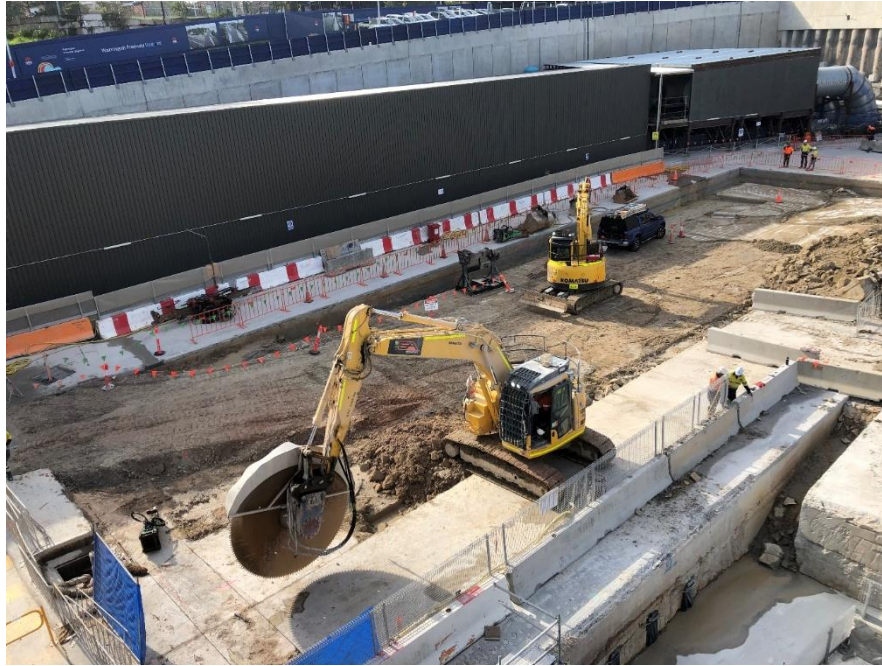
Figure 9. Saw cutting the trenches for building footings
