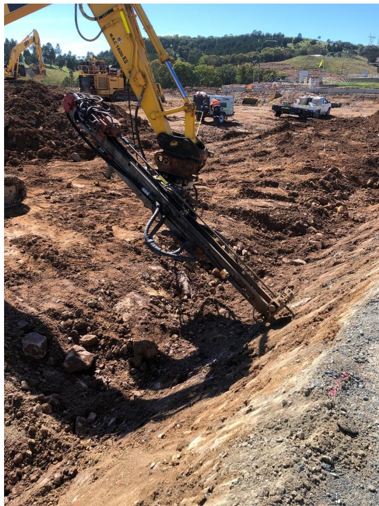
Figure 3 Drilling Soil nails
