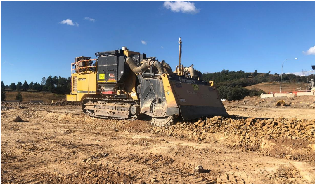
Figure 1. Excavation rock, 1255 Surface miner
